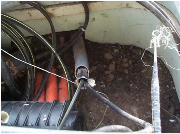
Fig. 8 Duct occupied with 2 resident cables
