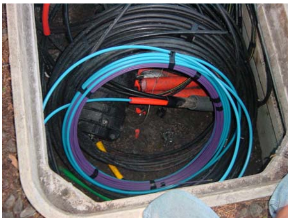
Fig. 10 Installed additional tube and cable
