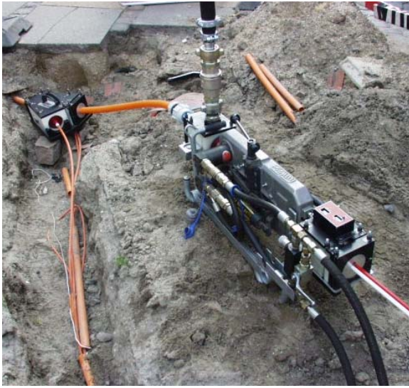
Fig. 12 Additional jetting Copenhagen
