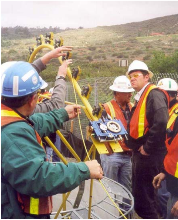
Fig. 4 Jetting microduct cables with buffering
