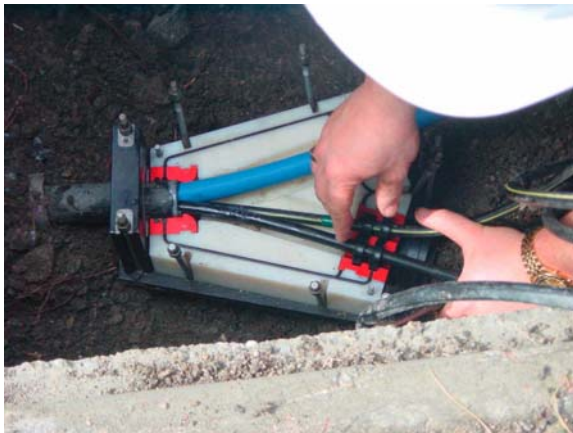
Fig. 9 Mounting Y-piece for additional jetting with 2 resident cables and guide for the tube
