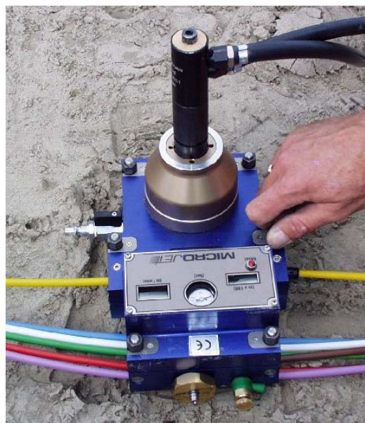
Fig. 3 Jetting microduct cables in tandem
