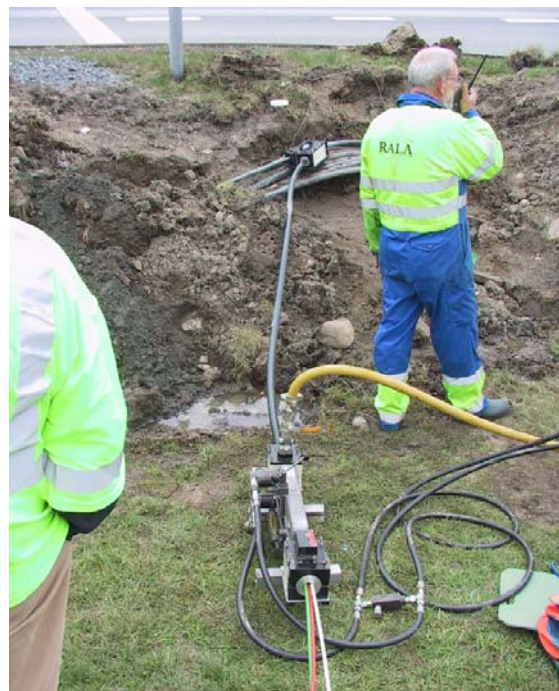
Fig. 11 Additional jetting of 3 tubes of 10 mm
